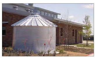
FIGURE 3.13 RAIN WATER COLLECTION SYSTEM Rain water collection system on a fire station in the dry climate of Denton, Texas. Source: Innovative Water Solutions, Austin, TX
