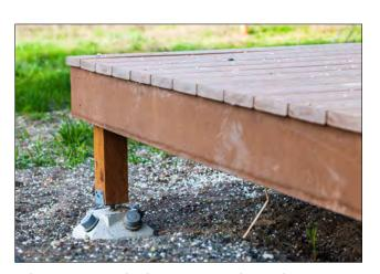
FIGURE **4.8.2** - USE OF MINIMAL EXCAVATION FOUNDATIONS FOR ACCESSORY STRUCTURES Deck constructed over piers.
