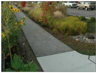
FIGURE **4.6.7**Pervious concrete.
