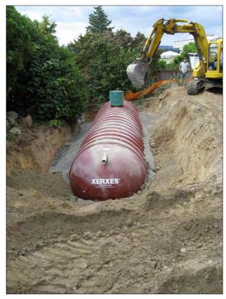
FIGURE **4.9.4** - EXCAVATION FOR AN UNDERGROUND CISTERN
