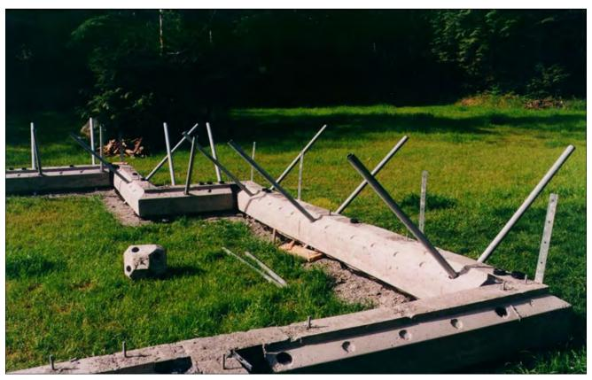
FIGURE **4.8.6** - WALL TYPE MINIMAL EXCAVATION FOUNDATION Pier type foundation. Source: Pin Foundations, Inc.
