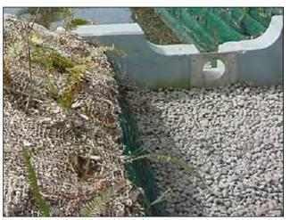
FIGURE **4.4.19**Aggregate mulch is used in the high gradient bioretention swale. Plants are installed through the aggregate mulch and into the BSM below.
