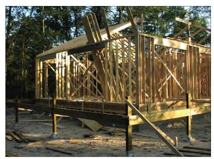
FIGURE **4.8.7** - FLAT SITE CONSTRUCTION ON PIERS Construction of a single-family home on piers on a relatively flat site Source: Pin Foundations, Inc.
