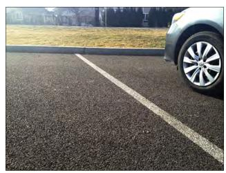
FIGURE **4.6.5**Porous asphalt at Yakima Kiwanis Park.
