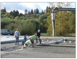
FIGURE **4.6.10**Hydraulically operated Bunyan screed compacts and provides the finished elevation in one preparation.
