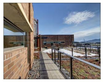
FIGURE 3.12 VEGETATED ROOF Benewah Medical Wellness Center vegetated roof, Plummer, Idaho. Source: NAC Architecture
