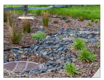
FIGURE **4.4.3**Arid climate bioretention example, Spokane.
