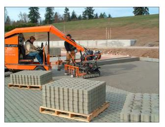
FIGURE **4.6.11**Mechanical paver installation.
