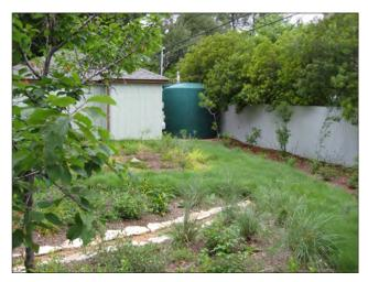
FIGURE **4.9.1** - POLYETHYLENE CISTERN Polyethylene cistern used to meet residential non-potable water demand.
