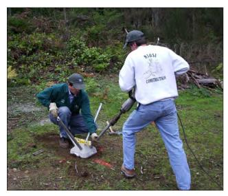
FIGURE **4.8.8** - PILE DRIVING Driving of pile with automatic hammer Source: Pin Foundations, Inc.
