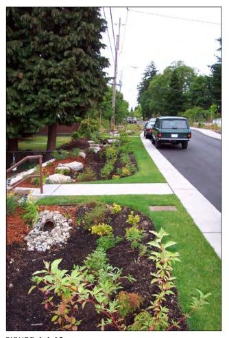
FIGURE **4.4.12**Bioretention area with flush curb and shoulder.
