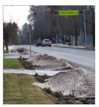
FIGURE **3.2** BIORETENTION SNOW STORAGE Snow storage in roadside bioretention in Spokane Source: AHBL, Inc. courtesy of Yakima Regional Low Impact Development Stormwater Design Manual
