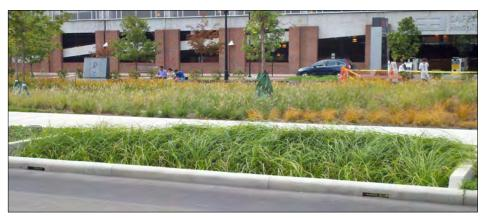
FIGURE **4.4.4**Bioretention in arid areas or other parts of the country, Columbus, Ohio. Source: AHBL, Inc.
