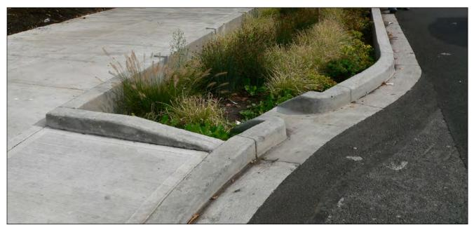
FIGURE **4.4.8**Typical curb cut details
