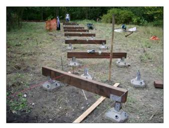
FIGURE **4.8.3** - FOOTBRIDGE WITH MINIMAL EXCAVATION FOUNDATION
