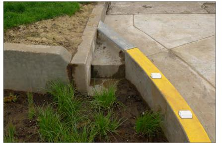
FIGURE **4.4.7**Curb cut inlet with drop to prevent clogging at flow entrance.
