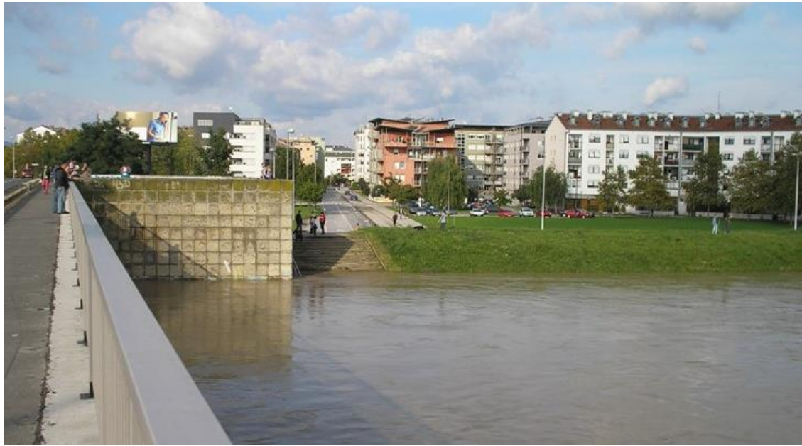
Figure 2.1.3. Embankment protecting Borovje from high water levels of Sava River
