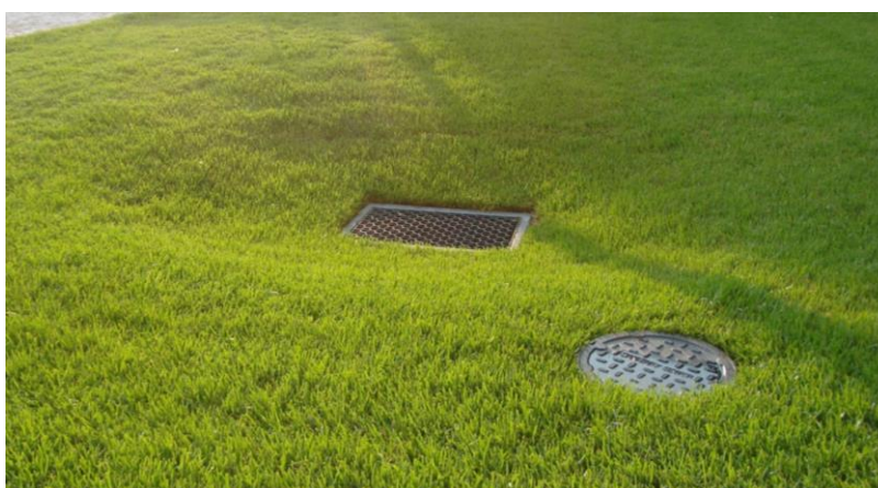
Figure 3.4.1.4 Park drain gutter
